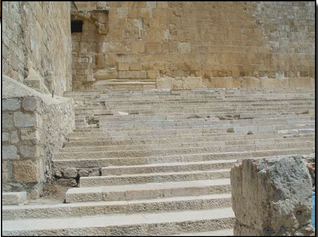
The remains of the steps leading to the Huldah Gate.
