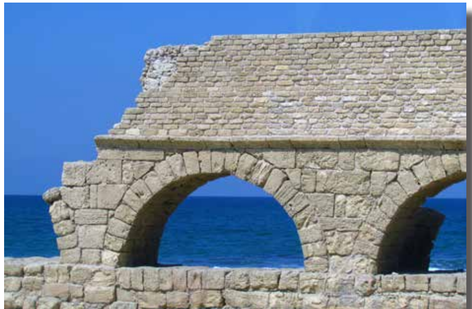
Caesarea was served by multiple aqueducts
