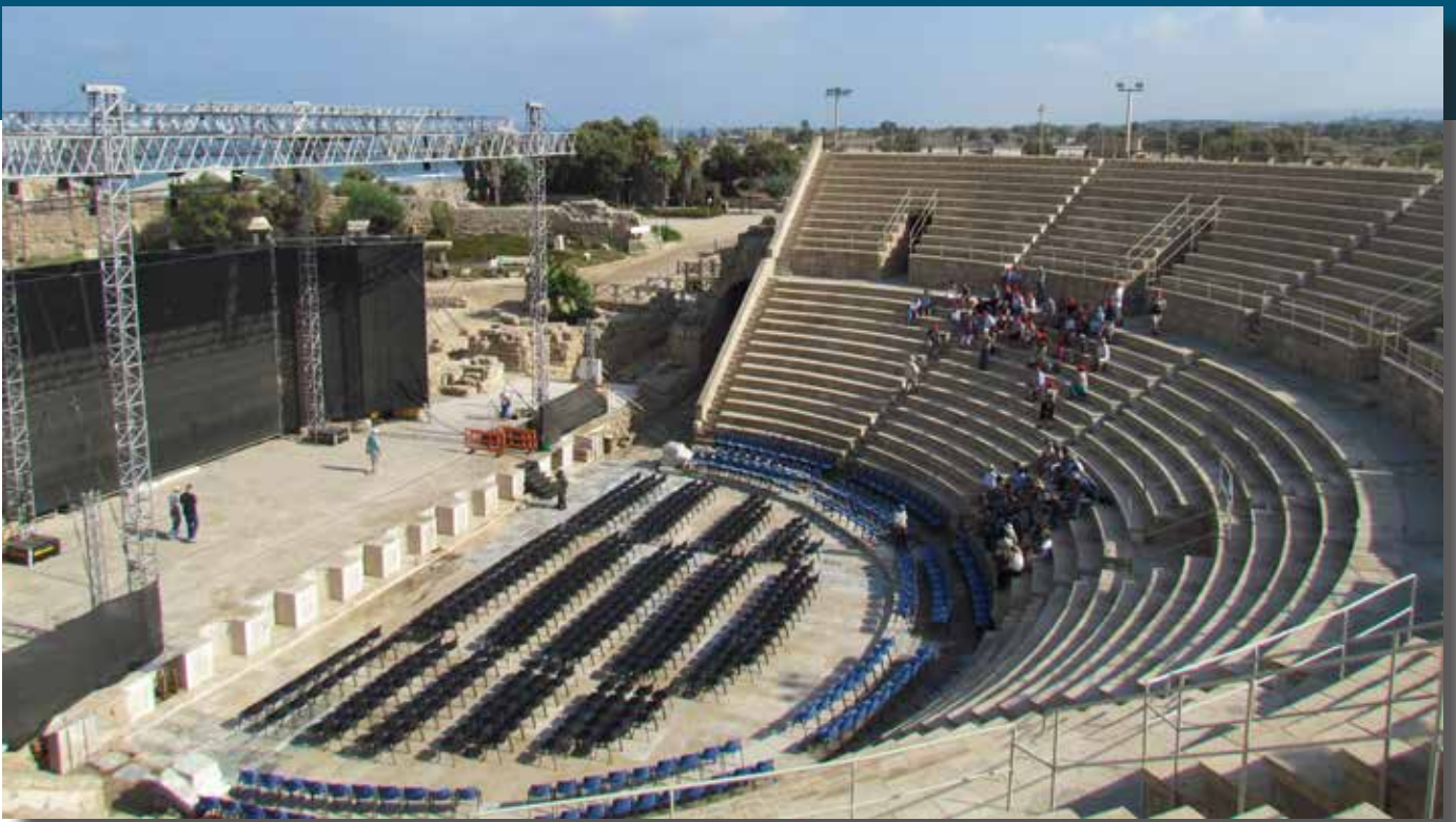
Theatre at Caesarea, reconstructed and occasionally configured for modern events, as shown here
