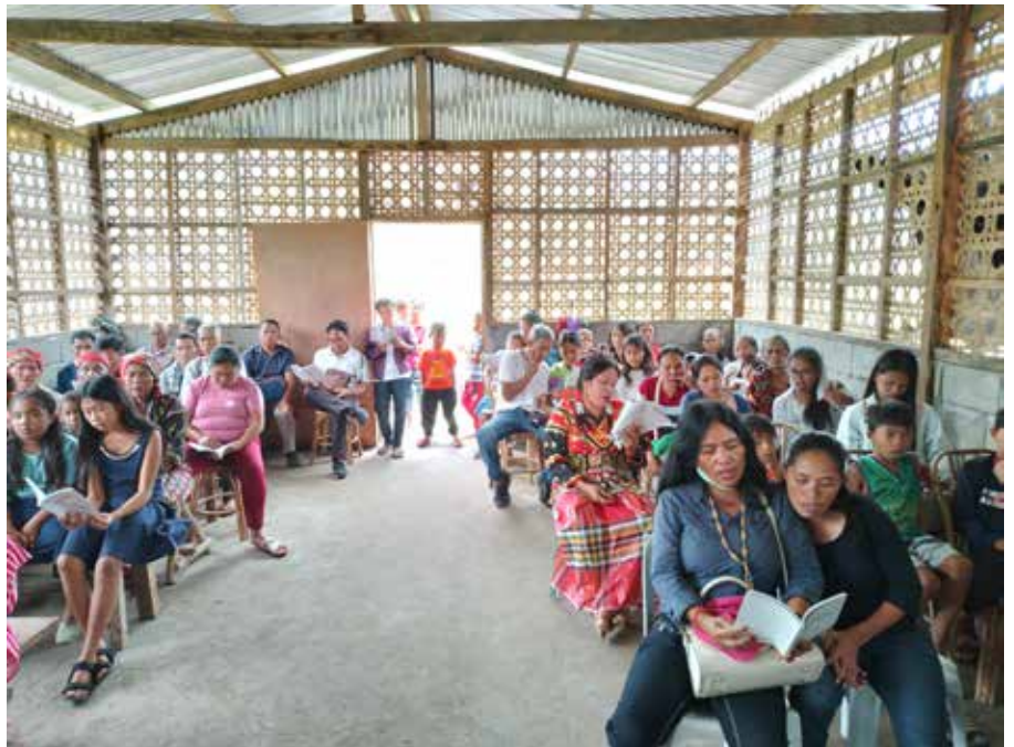
This newly constructed church building experienced a 5.9 magnitude earthquake for 30 seconds while I was preaching and remained intact and undamaged.
